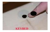
2. Drill a 3/8" hole through balance rail (preferably with a spade bit). Place action back in piano and mark position of this hole onto keybed below. Remove the action.
